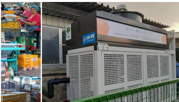
Fig. 7 Hydrocarbon refrigeration system installed in Province of Kotayk, Armenia
