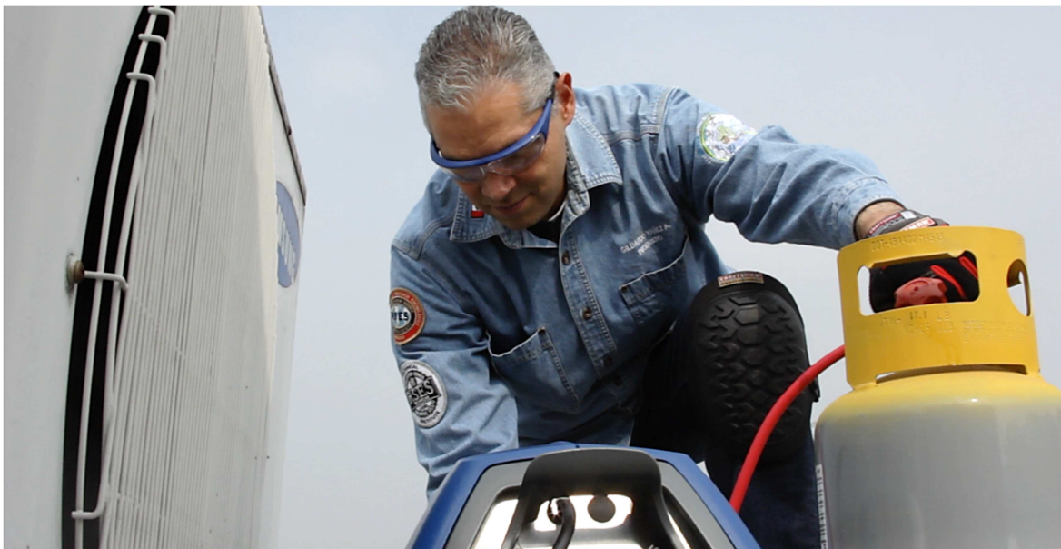
Figure 6 ODS recovery by Mexican servicing technicians
